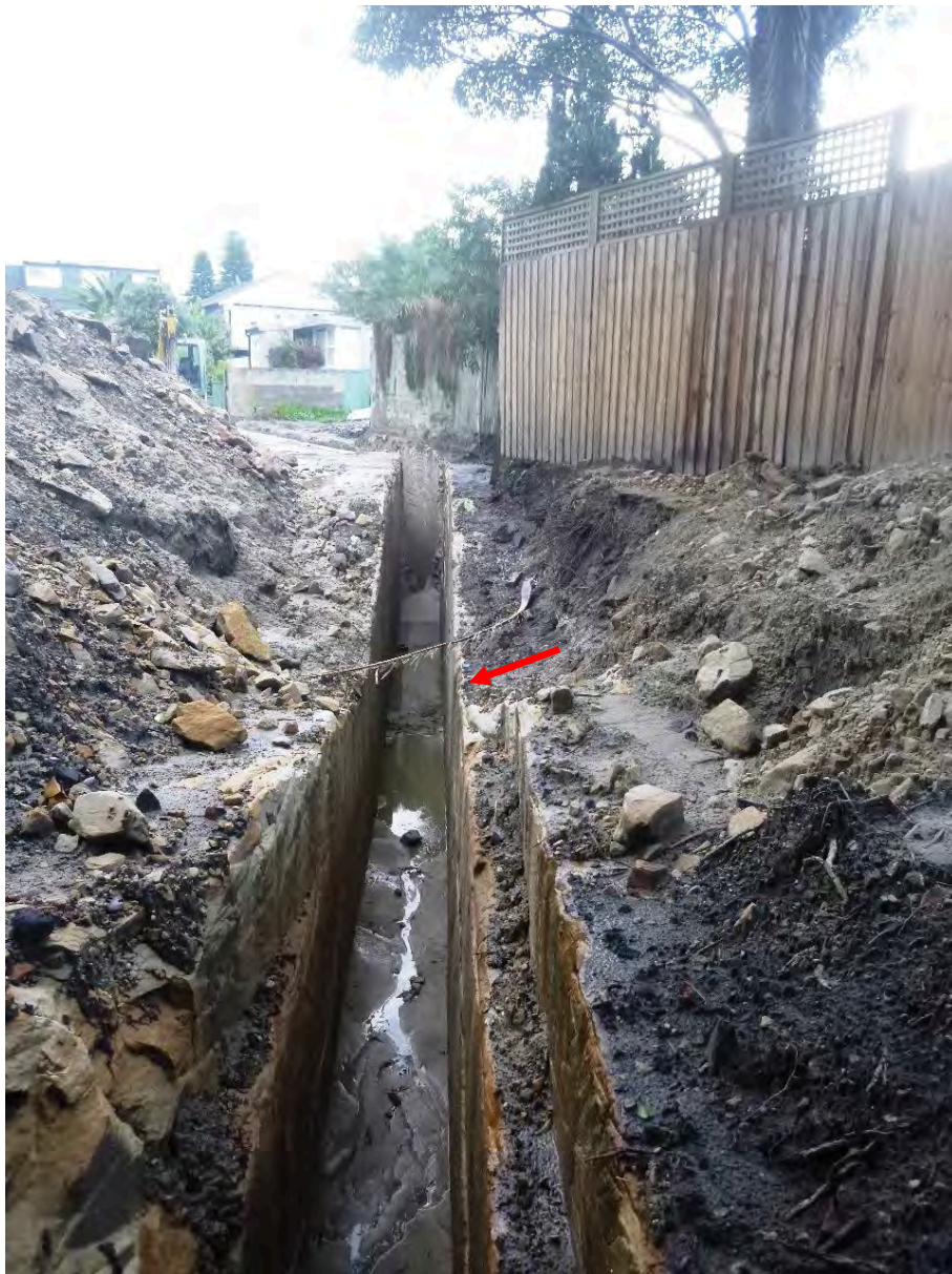
Historical Site Photograph of Sewer Diversion Trench, Photo 3 – View to south-west near Borehole BH5. Solid sandstone exposed at shallow depth along trench excavation. The approximate position of the clayey feature shown in Photo 4 is indicated as shown.
