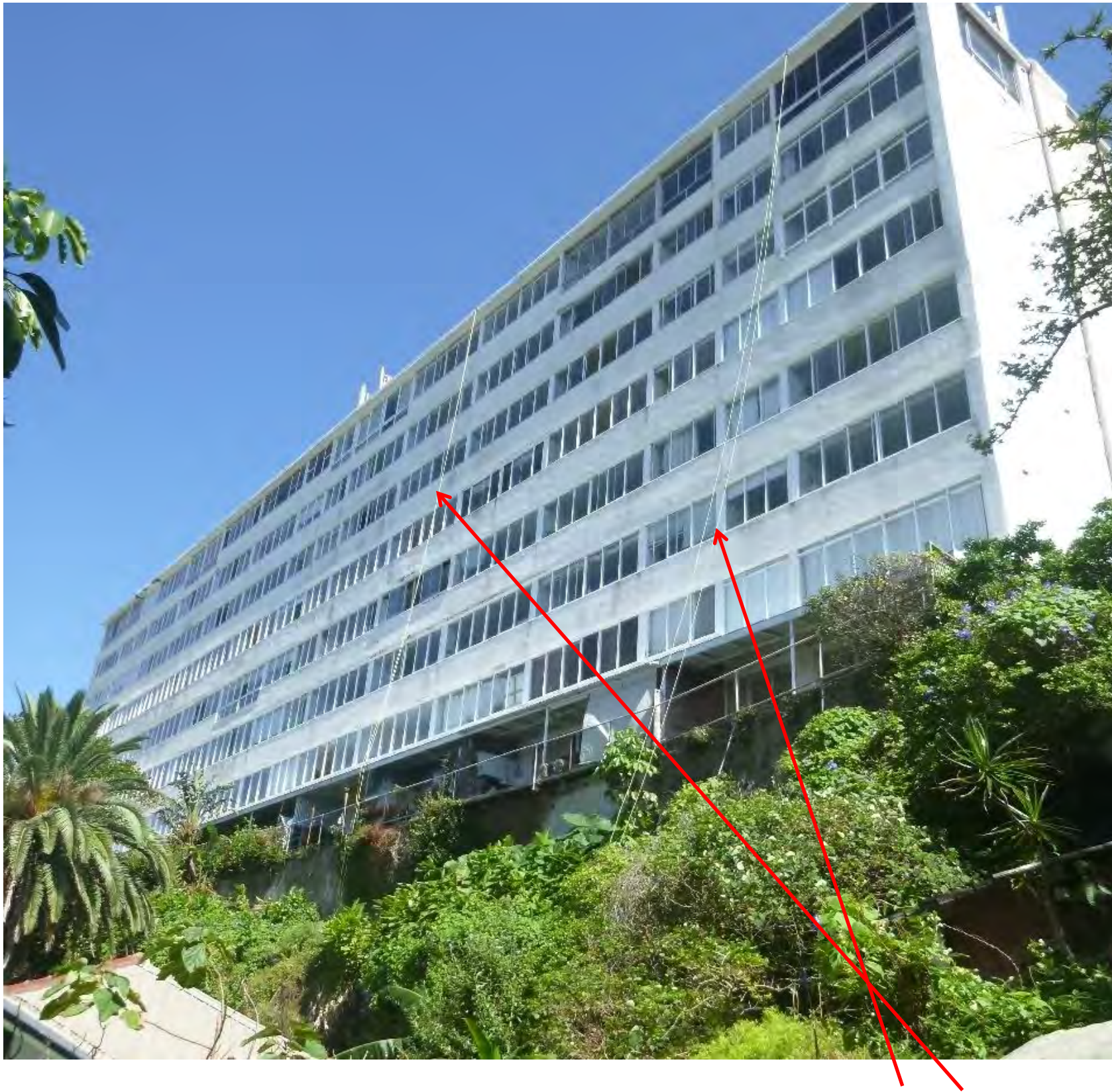
Photo 1. Southern side of building showing rope attachment locations to enable measurements for Cross Sections 1 and 2/3.
