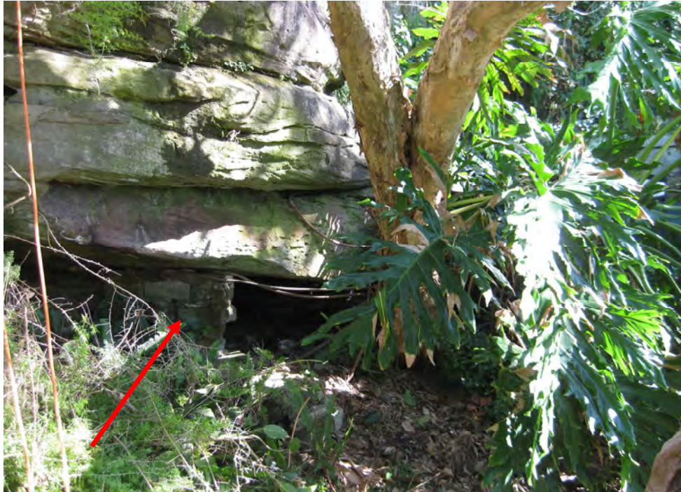
Mapping Traverse 105, Photo 4 – View towards traverse 104 from traverse 105. Overhang and cave formed within cross-bedded sandstone at toe of slope. Mortared brick underpinning observed within cave, indicated as shown.
