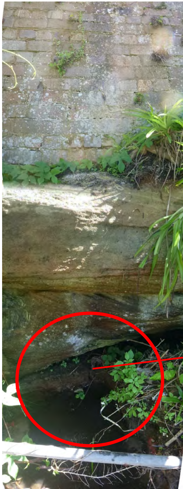
Photo 3. Cross Section 1; contact between brick terrace wall and sandstone bedrock showing lower very low strength rock.
