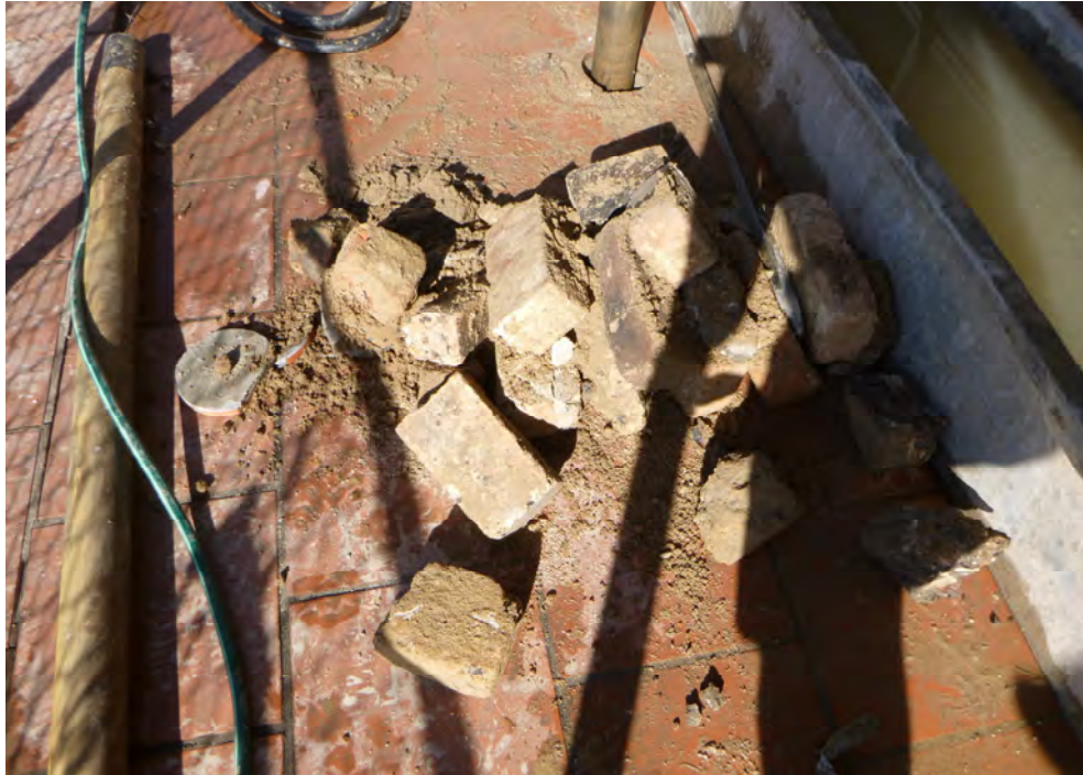
Photo D3 – View of rubble filling removed from Borehole BH206, drilled within the balcony of Unit 6.
