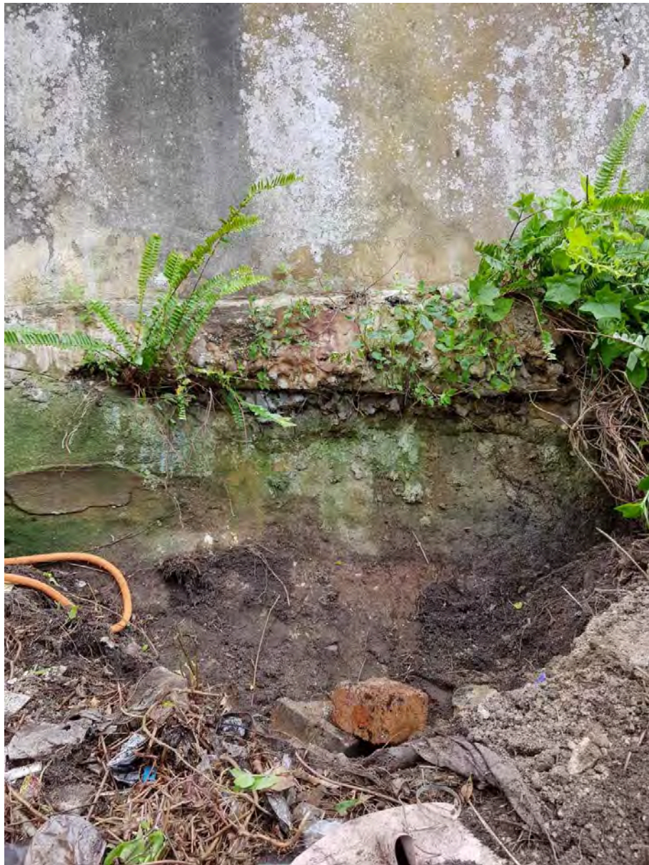
Mapping Traverse 102, Photo 1 – View of interface between rendered brick retaining wall and the underlying sandstone at mapping traverse 102, showing a thin layer of “levelling” concrete on top of the sandstone.
